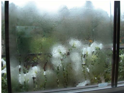
**Photo showing visual impact of external condensation on glass.<sup>4</sup>**
