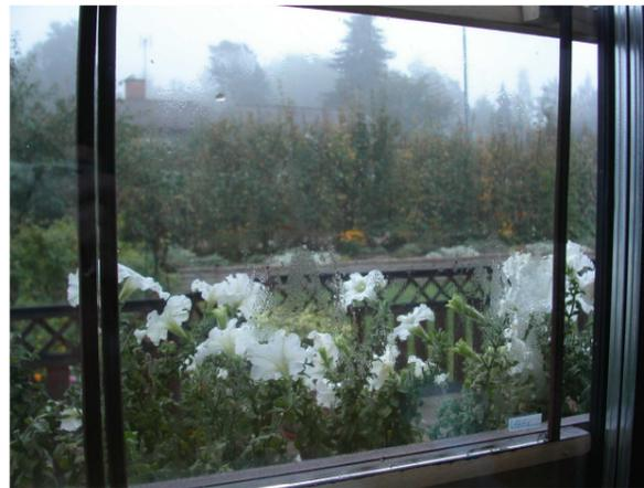
**Photo Showing Pilkington Activ™ With External Condensation. Note deterioration in visual impact is significantly reduced due to sheeting of water over surface.<sup>4</sup>**
